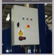
Electric panel available with speed adjustment, emergency stop relay and pre-start siren circuit
